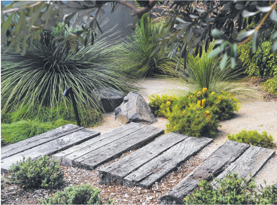
There's a four-metre drop from street level to the backyard which is managed by a series of level changes using railway sleepers and gravel.
